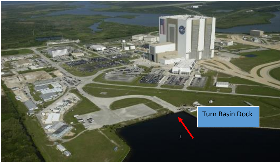
Kennedy Space Center's Turn Basin Dock (note Shuttle Landing Facility at top)
